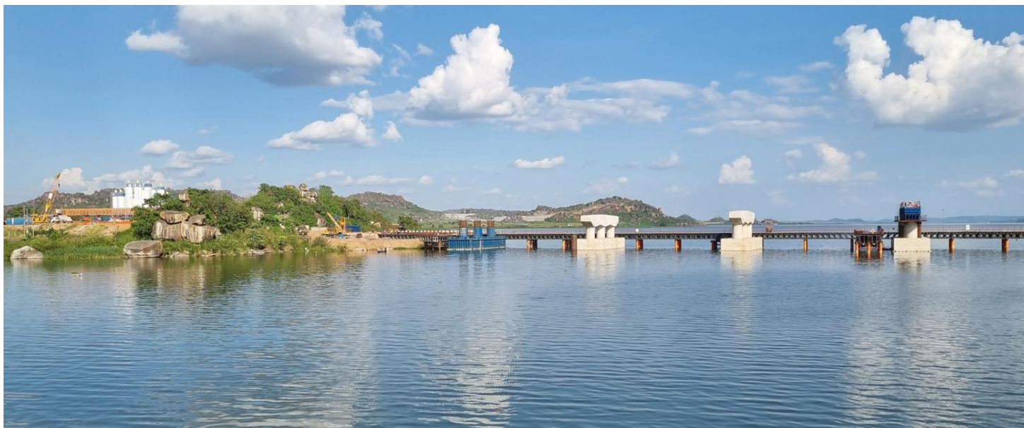
Figure 1: Bridge construction in progress
